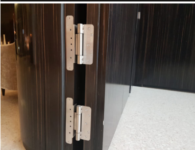
Caption 2: The barrel hinge system for the field of heavy-duty doors "Objecta" in use in the lobby of Grandhotel „The Fontenay“ in Hamburg: The huge door leaves with claddings are always open to an angle of 180 degrees and they will close automatically in the case of fire. Foto: BaSys
