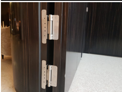
Caption 2: The barrel hinge system for the field of heavy-duty doors "Objecta" in use in the lobby of Grandhotel „The Fontenay“ in Hamburg: The huge door leafs with claddings are always open to an angle of 180 degrees and they will close automatically in the case of fire. Foto: BaSys
