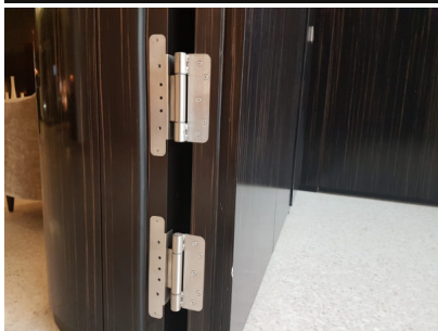
Caption 2: The barrel hinge system for the field of heavy-duty doors "Objecta" in use in the lobby of Grandhotel „The Fontenay“ in Hamburg: The huge door leaves with claddings are always open to an angle of 180 degrees and they will close automatically in the case of fire. Foto: BaSys
