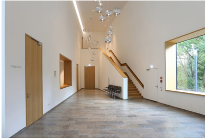
Caption 3: All interior doors in the Tauberphilharmonie Weikersheim are butt-mounted so that the door leaf is flush and harmonious with the frame and wall. Concealed hinges are discreetly discreet and allow the large-scale door design to work on its own. Photo: Michael Meschede, Kaufungen
