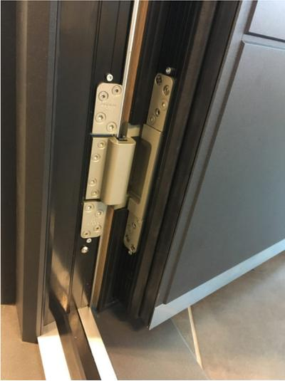
*Caption 1: Centrepiece of the Basys exhibition stand at the Fensterbau Frontale 2018 is the so-called "Winnerdoor", a wood and aluminium front door from the Italian Pradamano-based manufacturer Mixall. Fitted with "Masterband FX2 120 3-D FD", Basys is using this customer door to demonstrate how the technology can be adapted for concealed hinges on rebated house and apartment front doors with 18 mm rebate and door-leaf sealing. Photo: Basys*
