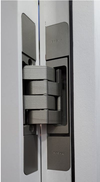
Caption 4: Basys presented a new solution to overcome claddings of up to 10 mm on both the frame and the leaf side with the "Pivota DX 110 3-D". Photo: BaSys
