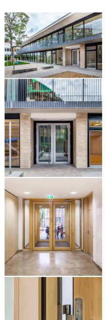
Caption: Heavy-duty door hinges from BaSys are used in the All Saints Kindergarten in Frankfurt. The double-leaf entrance door, a wood and aluminium construction, has four hinge systems for each door. The company Krebbers GmbH & Co. KG of Krefeld, used the "Objecta" hinges "2541/160/56-4" and the "Objecta" hinge retainers "STV 113/56 3-D" for a door weight of up to 160 kg (per pair). Photo: Daniel Vieser Architekturfotografie, Karlsruhe, www.dv-a.de
