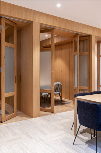
Caption 4: Three wooden frame glass folding walls – implemented using the “Hawa Varifold” folding/slide-in hardware – design the flowing transition to the three smaller units. They are made from glass so that daylight reaches the interior, while also providing privacy thanks to the opaque center section. When it is open, the partition wall discreetly retracts into a very small space thanks to the lateral suspension. When the partition walls are closed, a folding element designed as a hinged door secures the access to the smaller units. Photo: Hawa Sliding Solutions AG
